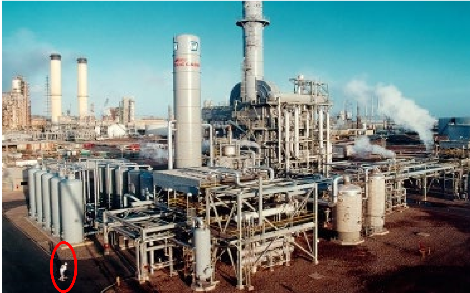
50 MMscfd Steam Methane Reformer Hydrogen Plant at Lagoven, Amuay in Venezuela
